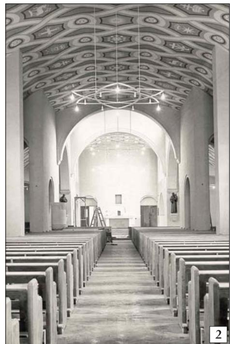
The ceiling was constructed of pre-cast concrete panels spanning between concrete purlins rendered and beautifully decorated to the designs of one of the Capuchins (*Fig 2*). The building was completed in the year of Goodhart-Rendel’s death (1959) and listed Grade II in 2008.
