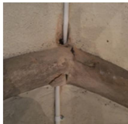
*An unfortunate route taken behind the hood mould of a window, damaging the stonework*
