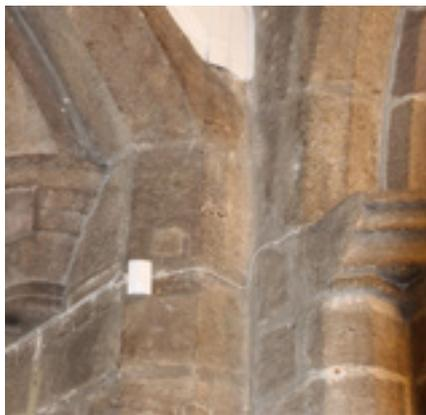
*These lead cables, redundant since 1975, have been cut back at the edge of the rendered area. Fixings remain in the stonework where the cables have been removed but the rendered wall surface would have been very badly damaged had all of the cables been removed.*
