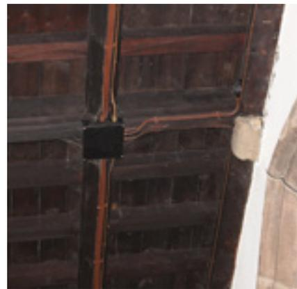
*Poor choice of cable route under an aisle ceiling: the junction box should have been fitted direct to the planking between the rafters with the cabling running along the top of the wall plate*
